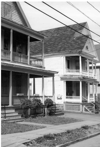
Fig. 31 Existing historic porches should be retained and carefully repaired. The design of replacement porches should be based upon solid physical or documentary evidence.
