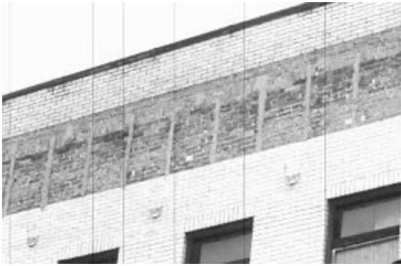
Fig. 9 As can be seen from the above, when a cornice is lost the result is devastating to the historic character of the individual building and of the streetscape.
