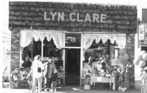
Fig. 11 Over the years, various renovation projects have resulted in the loss or obscuring of all historic materials on this nineteenth-century storefront. The latest application employed inappropriate treatments such as the use of artificial brick and a pent roof clad in wood shingles. Such rehabilitation treatments are not appropriate for the Utica Scenic and Historic District.
