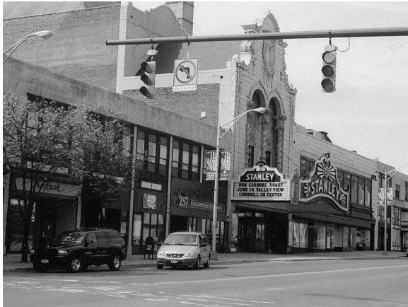
Utica's 1927 Baroque Revival-style Stanley Theater was built at a time when the moving picture industry had become firmly entrenched on the American scene.
