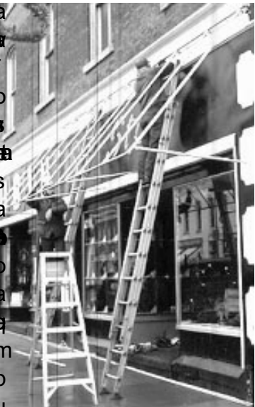
Fig. 40 The awning being installed here incorporates a system including a rigid pipe frame and a synthetic awning fabric. It is designed to remain extended throughout the year and employs a profile sufficiently sloped to assure that snow will not cause the structure to fail.
