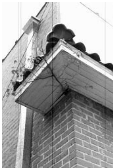
Fig. 28 If buildings and their individual components are not maintained regularly, deterioration will surely follow. In the photo above, dirt has accumulated in the gutter, encouraging the growth of unwanted and potentially damaging plant material.
