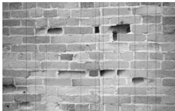
Fig. 17 When abrasive cleaning is undertaken, including treatments such as sandblasting or high-pressure water washing, spalling can occur to the soft brick surfaces of historic brick such as that found throughout Utica's Scenic and Historic District.
