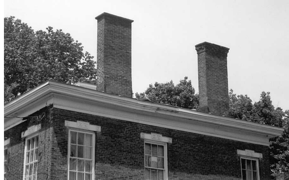
Fig. 30 Chimneys are significant architectural features and should be repaired and retained in any rehabilitation project.
