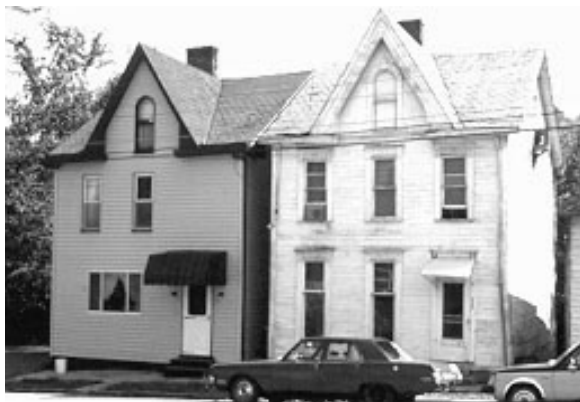
Fig. 23 As shown in the above photo of two identical houses, the installation of non-historic siding results in significant damage to the historic character of the building. Such treatment is not recommended in the Utica Scenic and Historic District.
