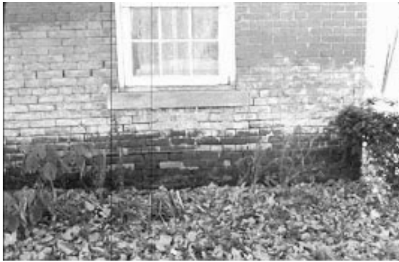
Fig. 20 The lack of an adequate drainage system has created serious problems for this historic brick building, including the growth of moss on the sides, the penetration of moisture into the surfaces, and the accelerated deterioration of the brick and mortar. This problem can occur on residential or commercial buildings of wood or masonry construction.
