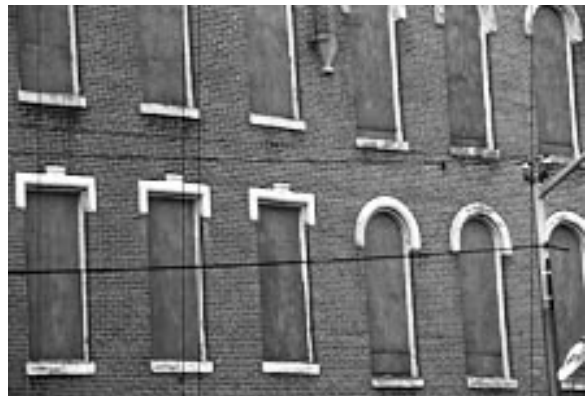
Fig. 25 Whether space is vacant or fully-utilized, windows should always be maintained in good condition, without broken panes or deteriorated trim. The boarding up of windows should not occur within the Utica Scenic and Historic District.
