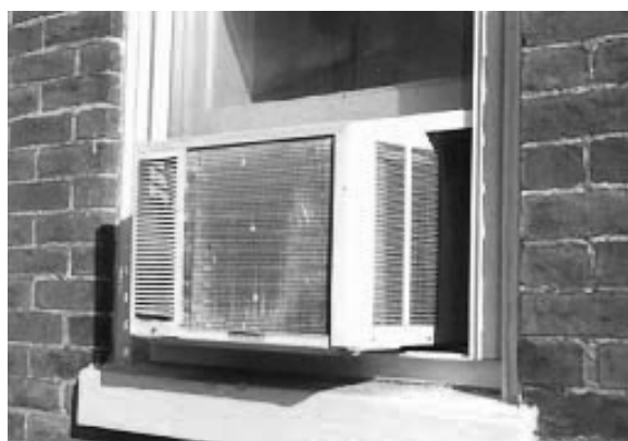
Fig. 27 Window air conditioners should be installed only on secondary elevations--preferably on the rear or side of a building--and should never damage historic building materials.
