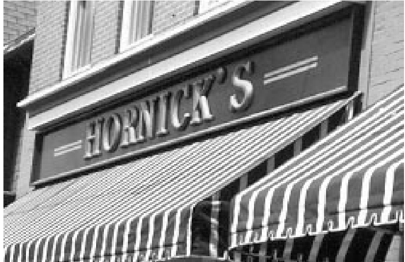
Fig. 37 Only in selected instances is the use of synthetic materials appropriate within the district. One such example is depicted above in the synthetic awning fabric and the plastic letters which were employed in this very successful storefront rehabilitation project.
