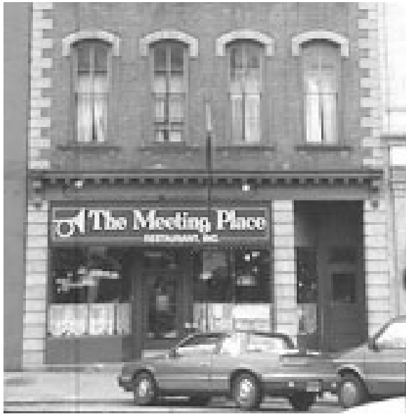
Fig. 33 The signage for this commercial building was carefully chosen and was executed in a manner consistent with the historic commercial character of the property, including the installation of a flat-mounted sign within the upright storefront piers and inside the signband designed for that particular storefront.
