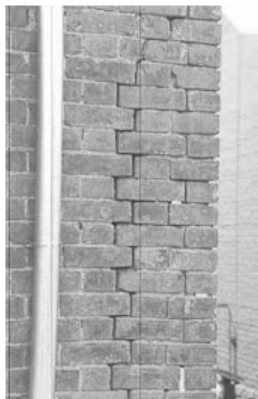
Fig. 29 The new half-round downspout shown above was installed well after the lack of proper drainage had caused failure in the corner of this historic brick building. Proper guttering and water diversion systems should be well-maintained throughout the Scenic and Historic District.
