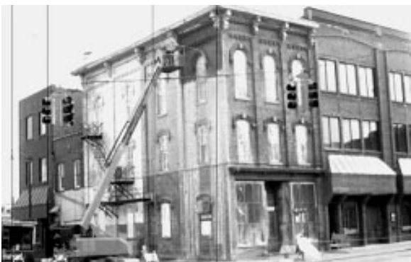
Fig. 14 The process of cleaning a painted historic building involves both the stripping of paint and cleaning of dirt which has accumulated on the surface.
