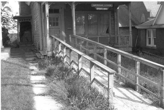
Fig. 42 The unpainted pressure-treated wood ramp on this small historic building extends completely to the sidewalk, impacting negatively on the streetscape. It appears to be of poor quality construction and is visually incompatible with the character of the building.
