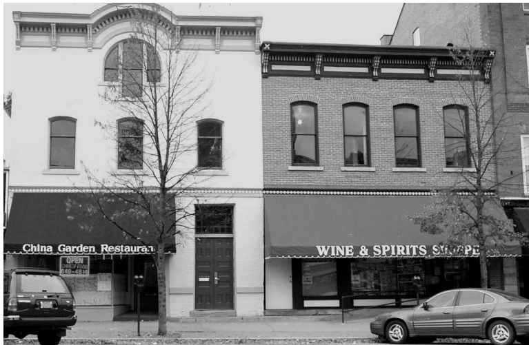
Fig. 39 These two buildings illustrate the use of stationary awnings whose location and graphics have been selected with great care. The use of such design solutions is encouraged for buildings throughout the Scenic and Historic District
