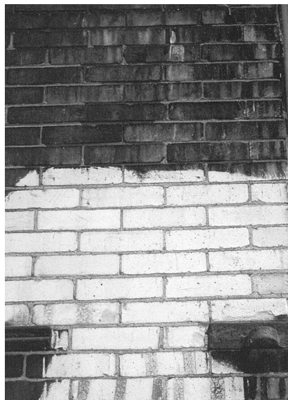
Fig. 16 A test patch taken prior to a cleaning project will confirm whether or not a building is a candidate for such rehabilitation activity.
