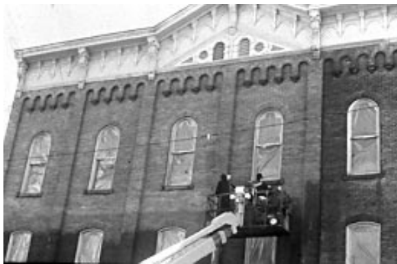
Fig. 13 The cleaning of this previously-unpainted 1880s building demonstrates the dramatic visual effect of properly executed masonry cleaning. Using an environmentally-acceptable cleaning solution and a low-pressure water rinse, the surfaces were cleaned without any repointing being necessary.
