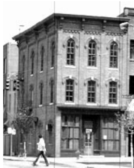
Fig. 15 When paint is stripped from a historic building, not only must care be taken not to harm the brick and mortar, but the residue must be collected and disposed of in an environmentally-responsible manner (see Fig. 14, left). As shown in the "after" view, above, the results are impressive.
