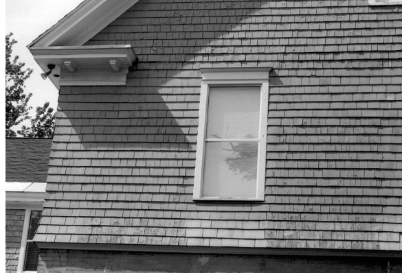
Fig. 22 This Genesee Street home exhibits shingled wall surfaces which provide a very distinctive "skin" for the home. Such surfaces should always be repaired and should not be covered with non-historic materials.
