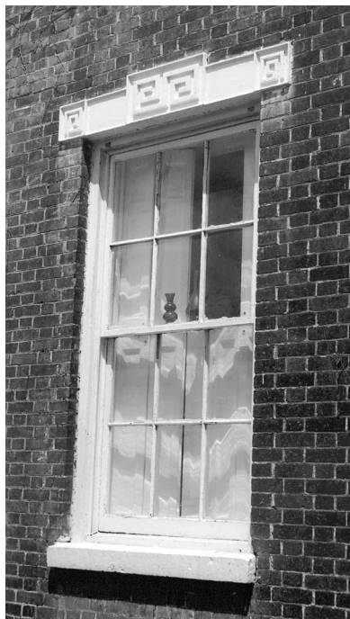
Fig. 26 This handsome six-over-six-light window dates from before the Civil War and retains the small-paned windows characteristic of the era. Such sash should generally not be used on homes dating from the late 1800s and beyond, unless their historic presence can be documented.
