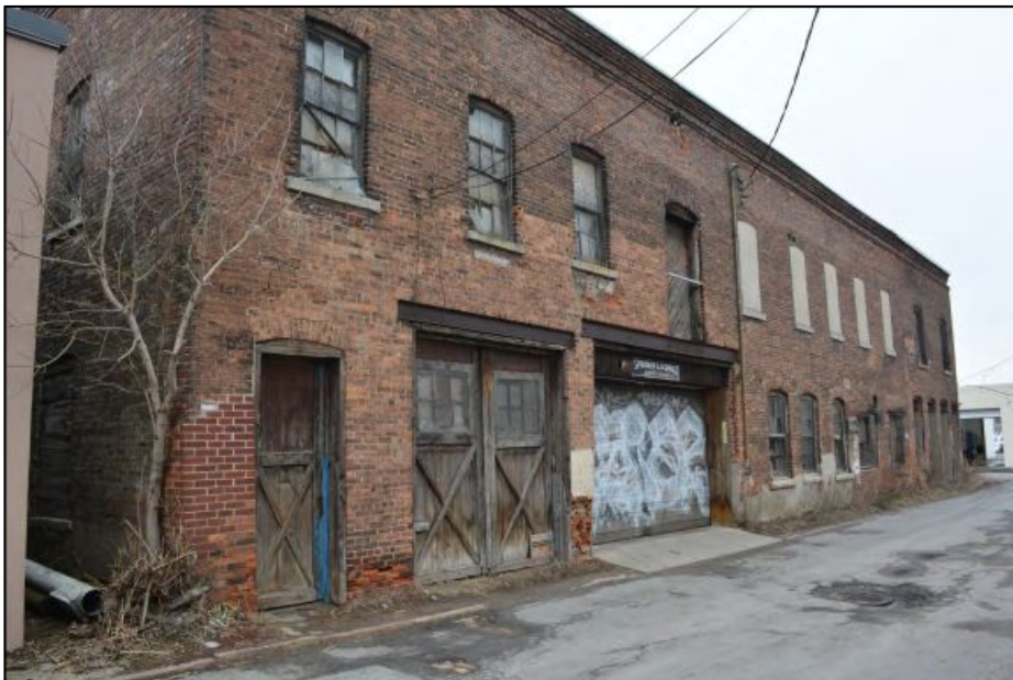
Figure 14. 529 Oriskany Street Looking Northeast
