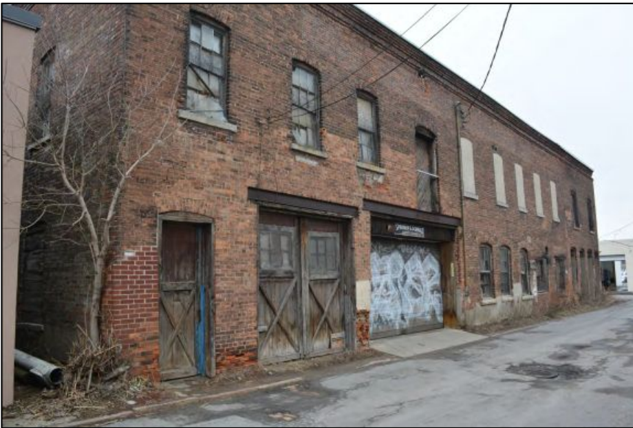
Figure 23. 529 Oriskany Street Looking Northeast
