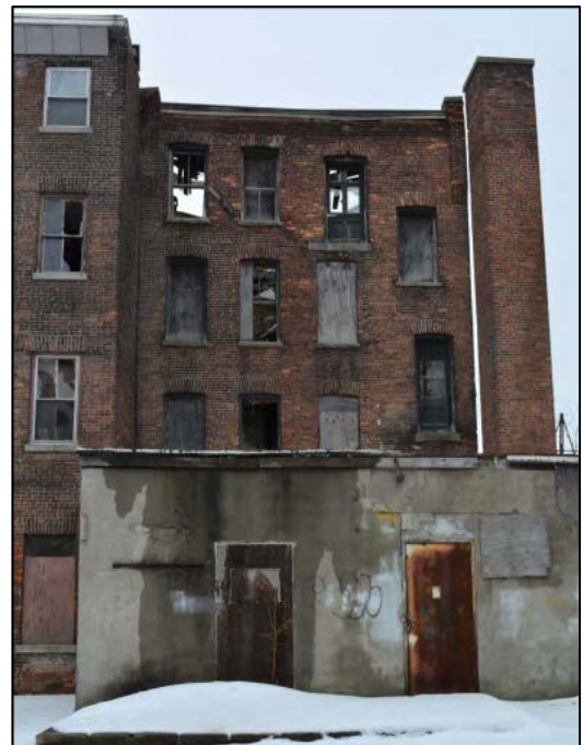
Figure 15. 336 Columbia Street Facing South
